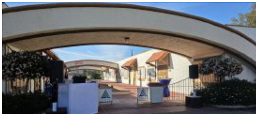
Built in 1977, the Powell Building formerly housed office professional tenants.
